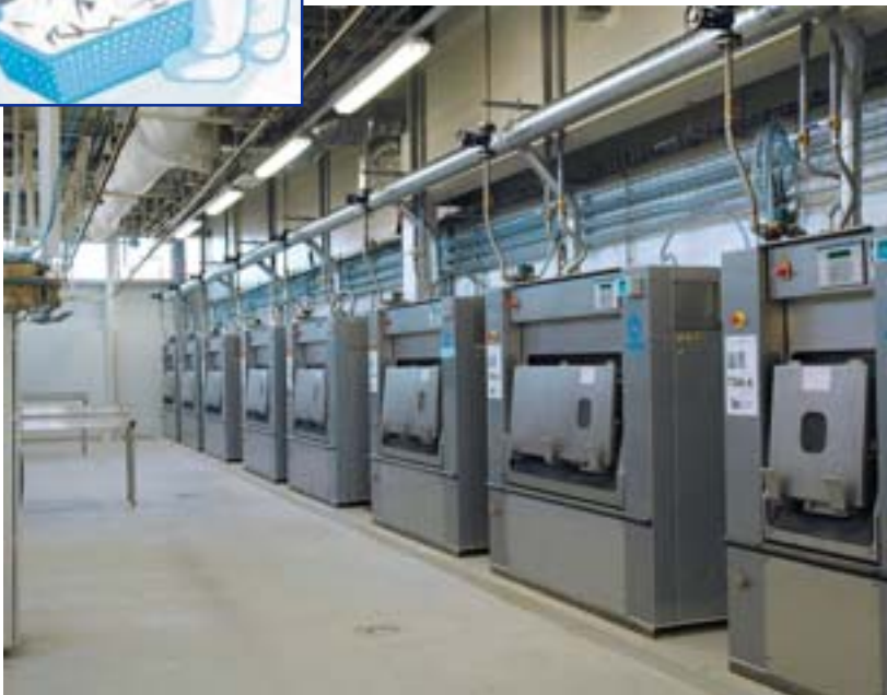
Dual opposed doors, separated by a sanitised partition, prevent cross contamination
